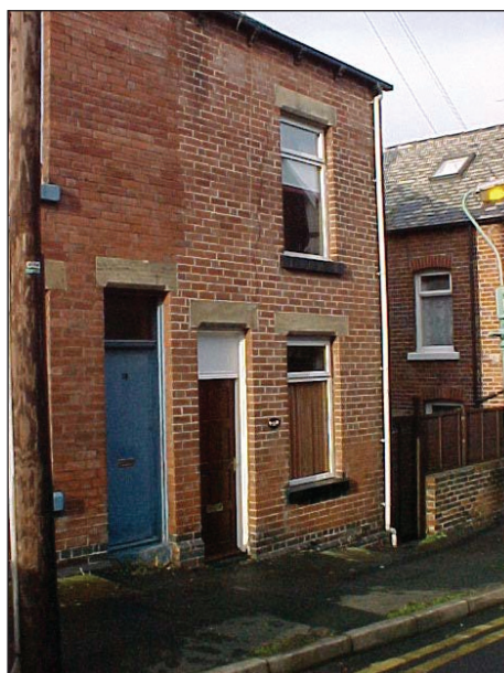
Narrow frontage house Dwelling: pre-1920 mid-terraced
